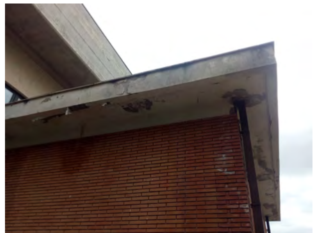
Cornicioni in c.a.
